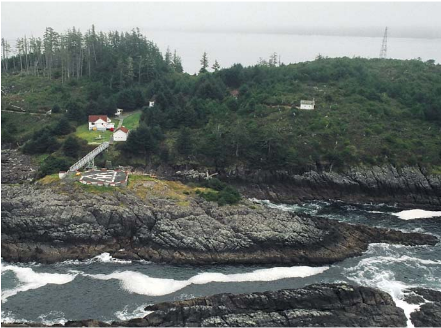
Egg Island Lightstation, on the edge of Queen Charlotte Sound near Cape Caution, on B.C.'s mainland central coast. Its light is atop the tower at right. The helipad is the former site of the actual lightstation, destroyed by storm wind and 25-metre seas in 1948 in which there were no fatalities. The station is still staffed.
